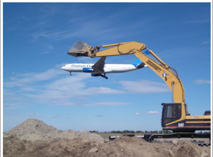
Calgary International Airport EllisDon Construction Management
